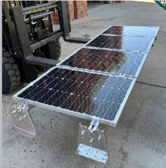
Top to bottom: Build on Floor installation method, Build on Roof installation method, Build on Floor assembly hoisted up by forklift
